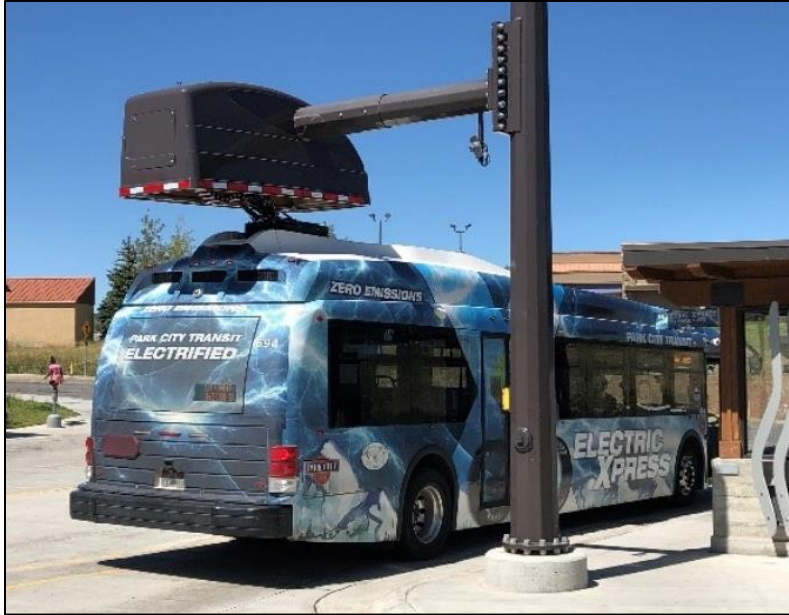
Figure 22: Example of On-Route Quick Charging
