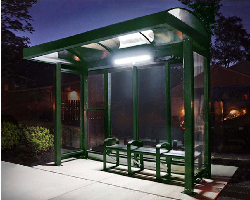
Figure 20: Example of a Public Bus Stop with Safety Lighting
