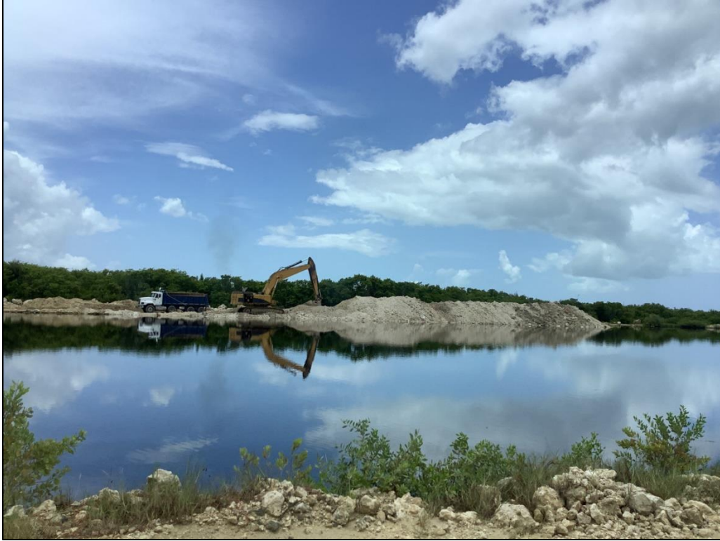
Figure 15: Active Quarry (July 2023)
