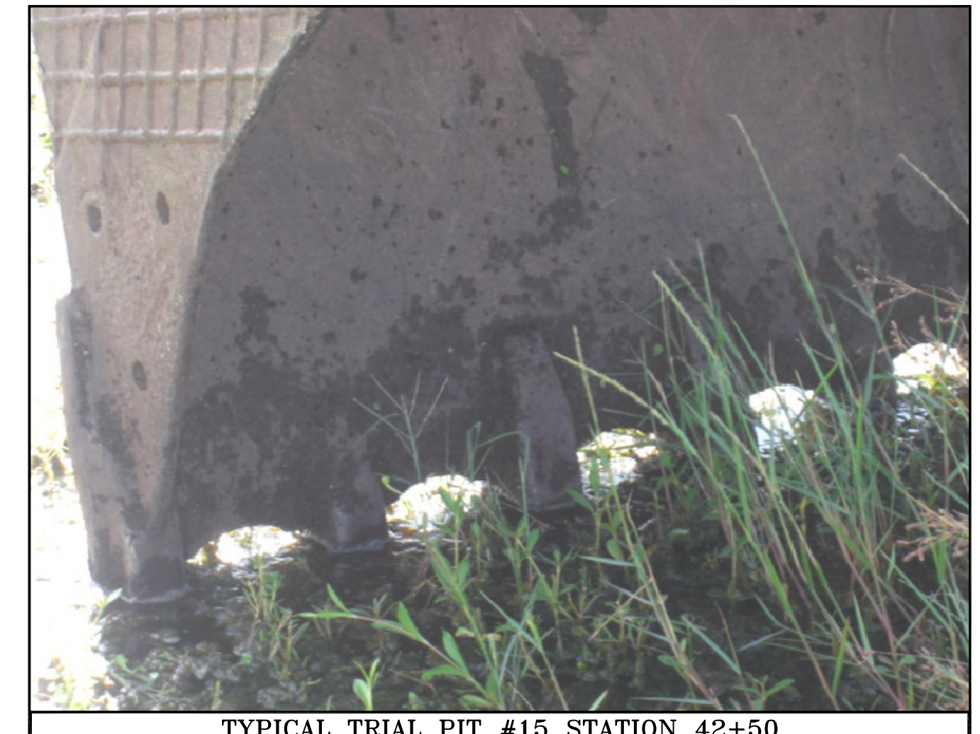
TYPICAL TRIAL PIT #15 STATION 42+50
