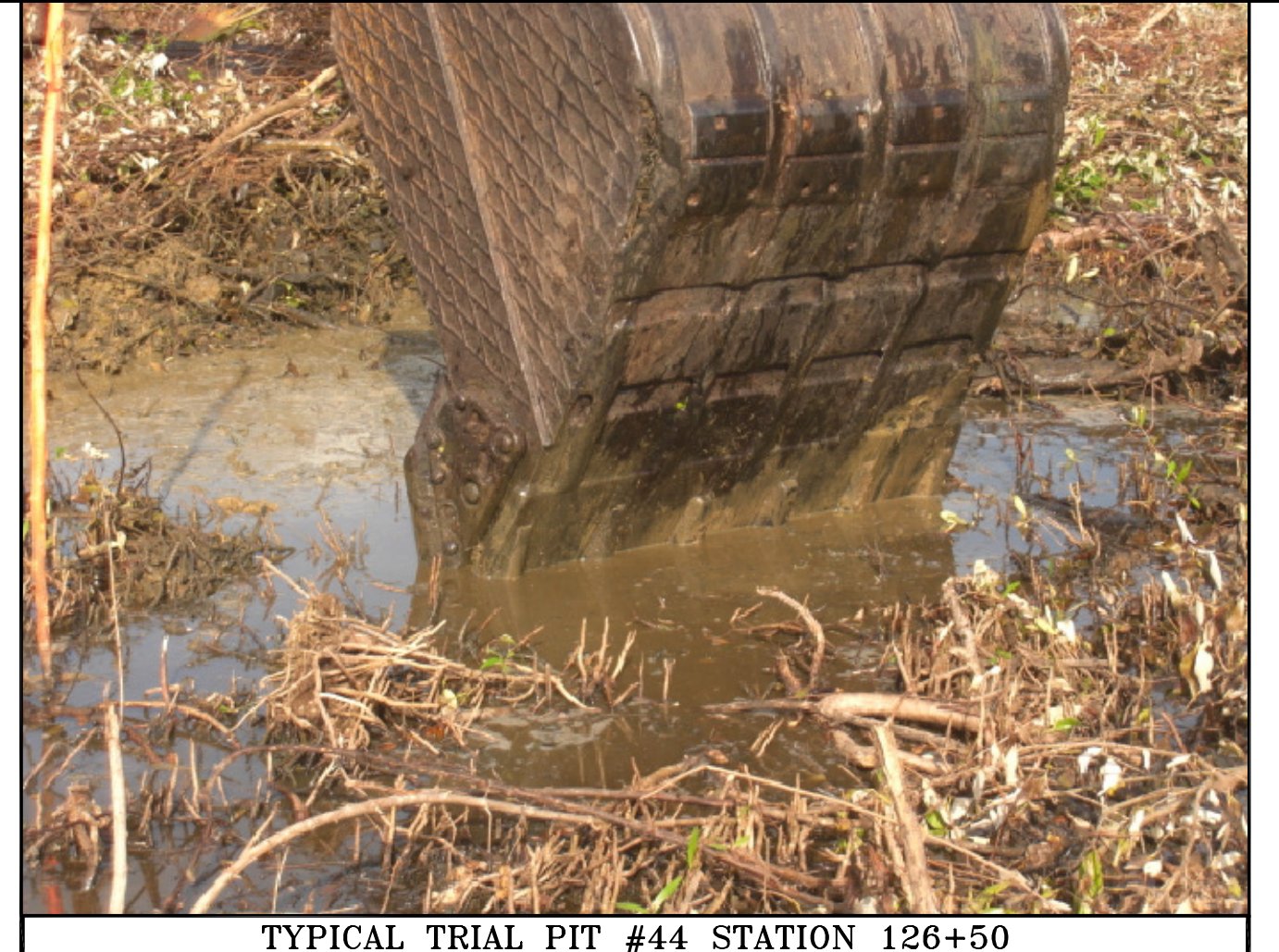
TYPICAL TRIAL PIT #44 STATION 126+50
