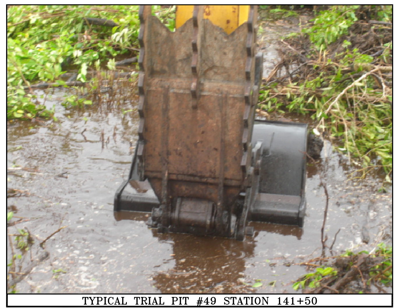
TYPICAL TRIAL PIT #49 STATION 141+50
