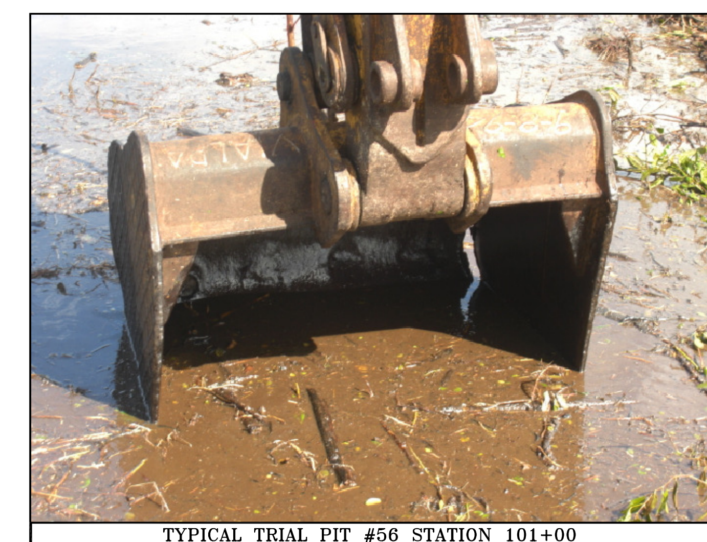
TYPICAL TRIAL PIT #56 STATION 101+00
