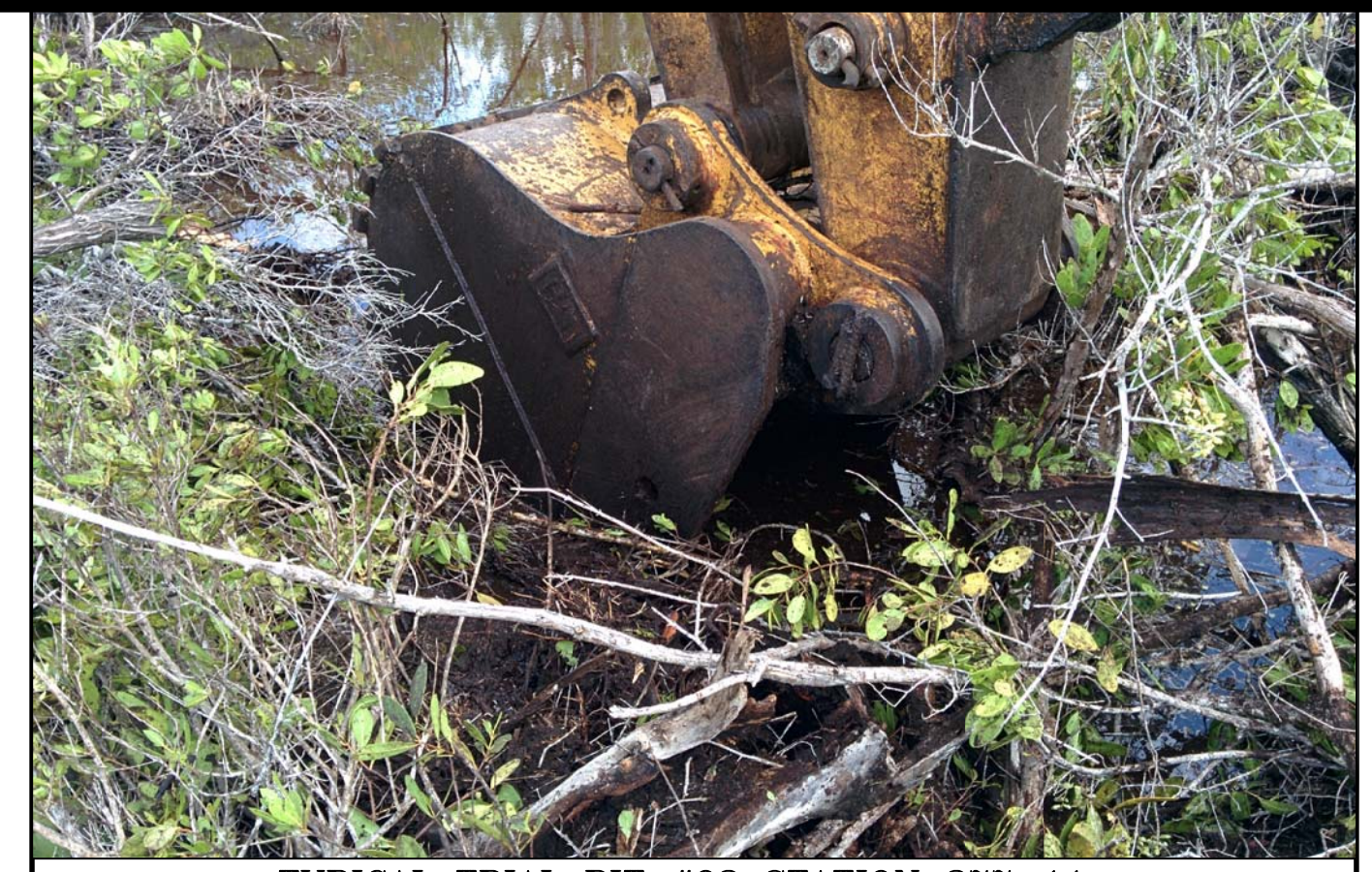
TYPICAL TRIAL PIT #92 STATION 277+11
