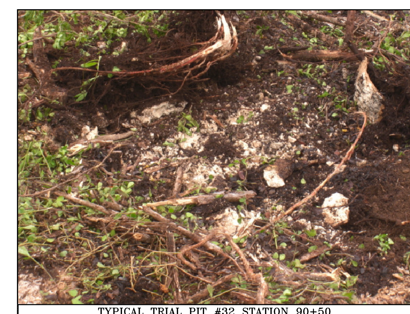
TYPICAL TRIAL PIT #32 STATION 90+50
