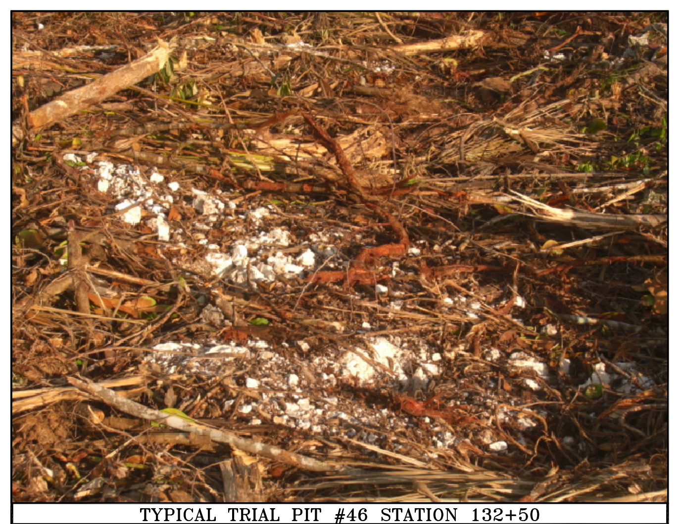
TYPICAL TRIAL PIT #46 STATION 132+50
