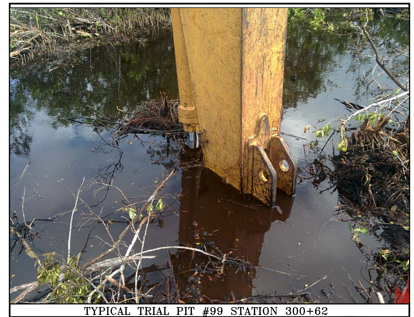
TYPICAL TRIAL PIT #99 STATION 300+62
