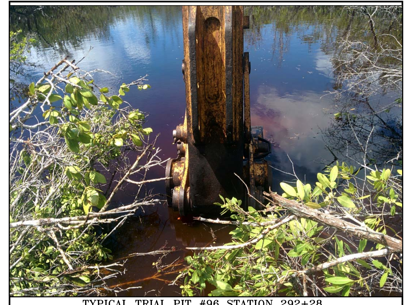
TYPICAL TRIAL PIT #96 STATION 292+28
