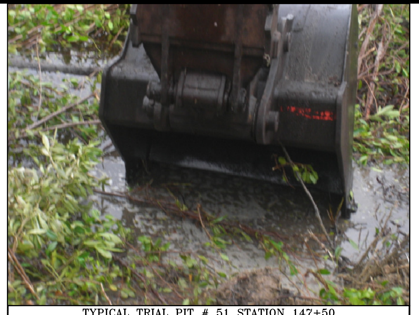
TYPICAL TRIAL PIT # 51 STATION 147+50
