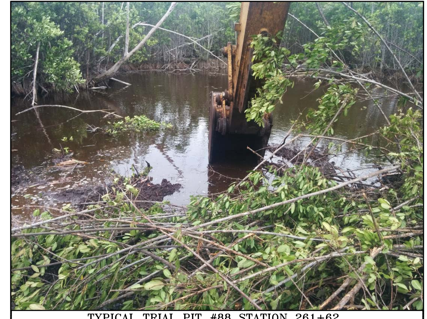
TYPICAL TRIAL PIT #88 STATION 261+62
