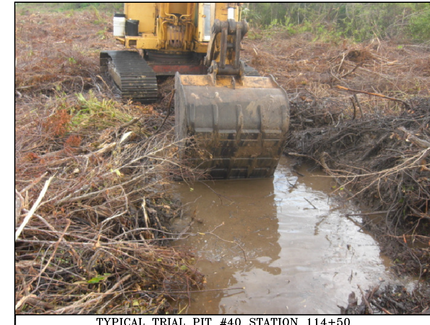
TYPICAL TRIAL PIT #40 STATION 114+50
