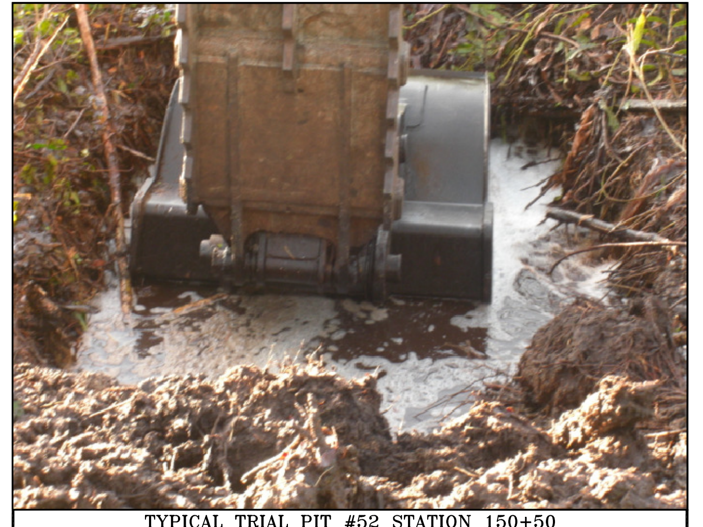
TYPICAL TRIAL PIT #52 STATION 150+50
