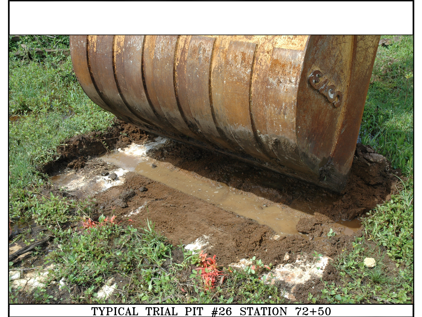
TYPICAL TRIAL PIT #26 STATION 72+50
