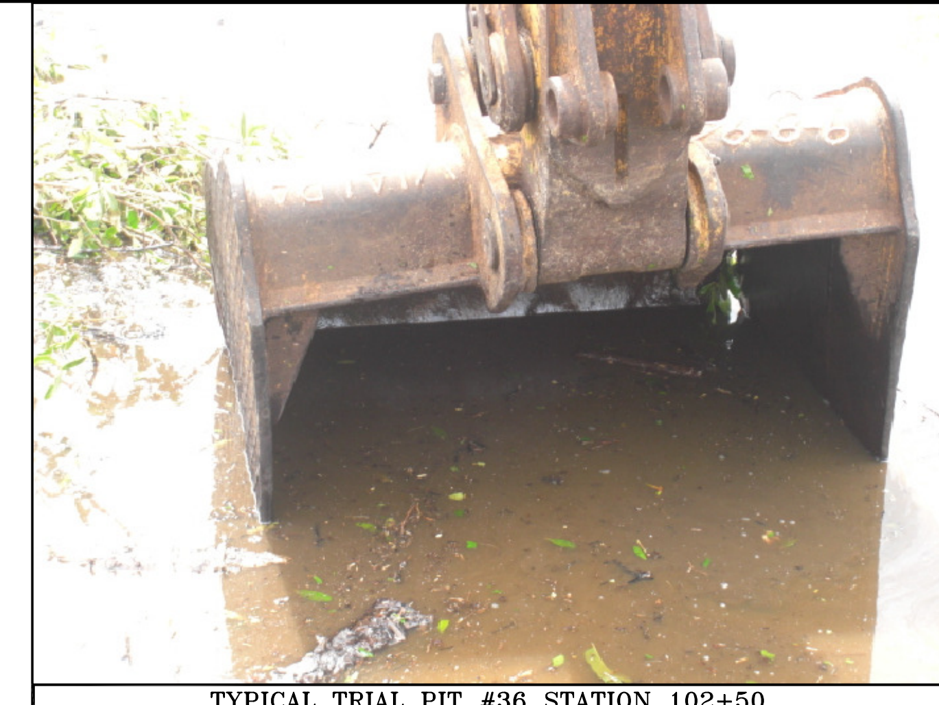
TYPICAL TRIAL PIT #36 STATION 102+50
