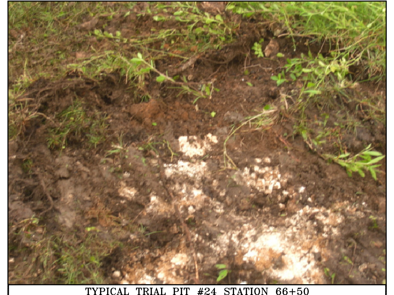
TYPICAL TRIAL PIT #24 STATION 66+50
