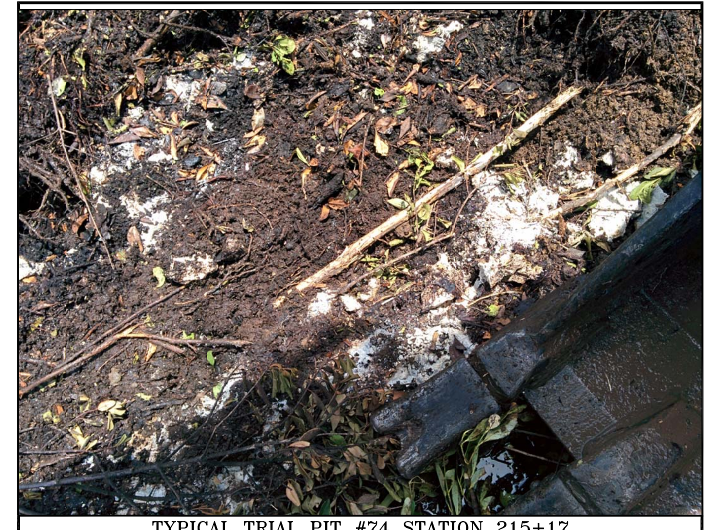
TYPICAL TRIAL PIT #74 STATION 215+17
