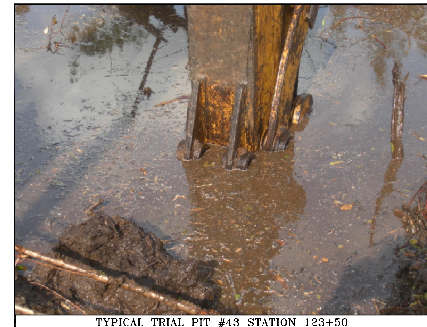
TYPICAL TRIAL PIT #43 STATION 123+50
