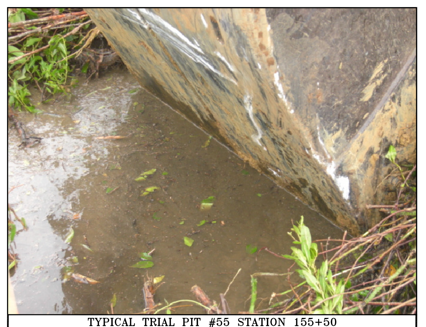
TYPICAL TRIAL PIT #55 STATION 155+50
