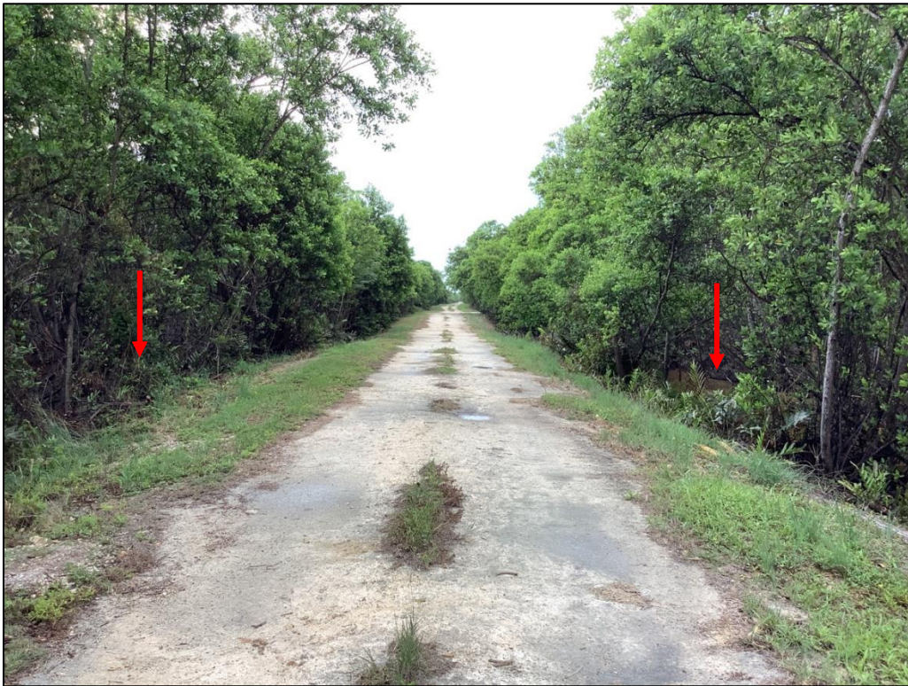
Photo 15: Access road with adjacent mosquito ditches (July 2023)
