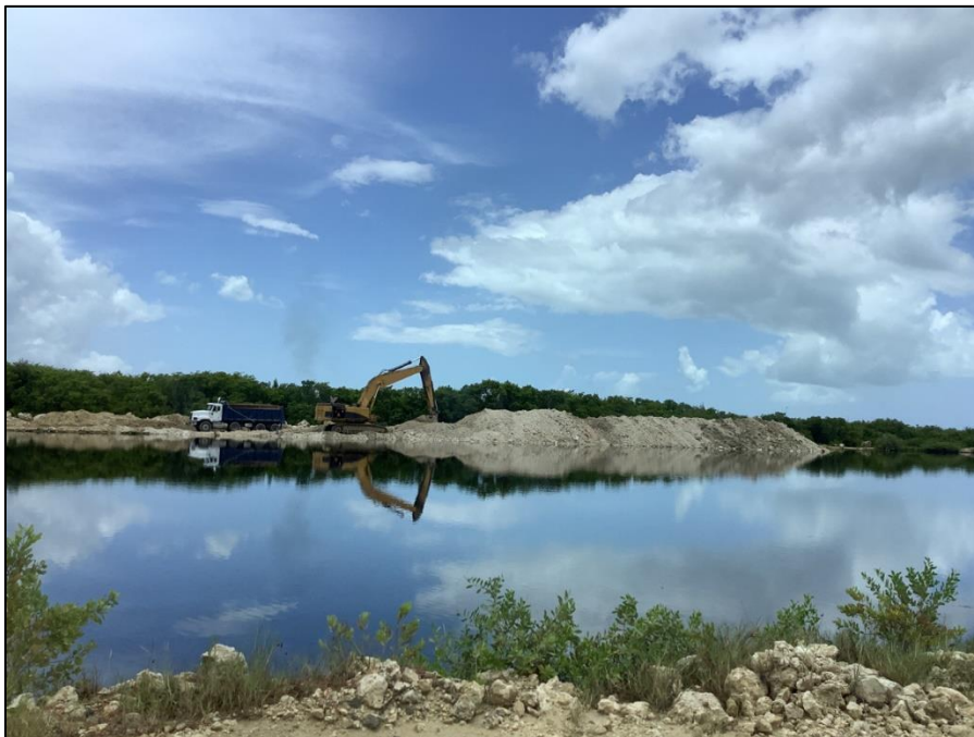
Figure 13: Active Quarry located northeast of Meagre Bay Pond (July 2023)
