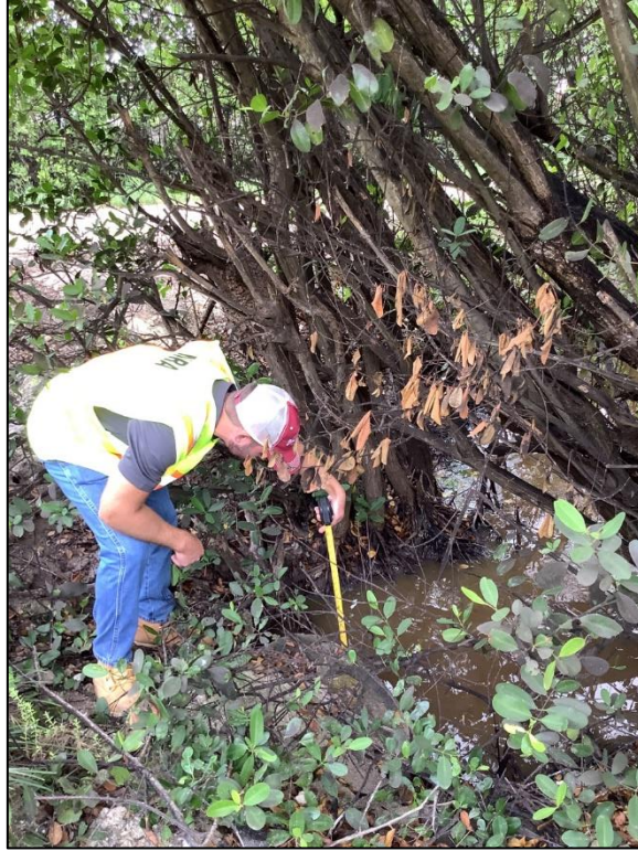
Photo 16: RCP drainage pipe (July 2023)
