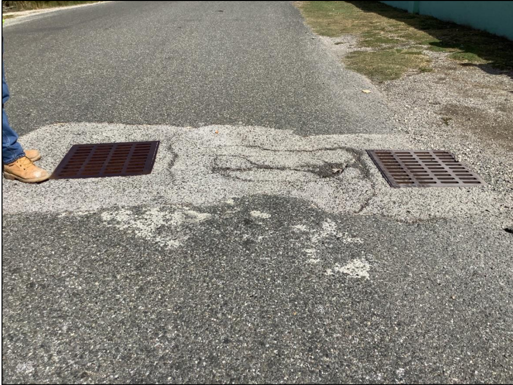
Photo 4: Inlet on shoulder drains to inlet in centre of roadway (July 2023)
