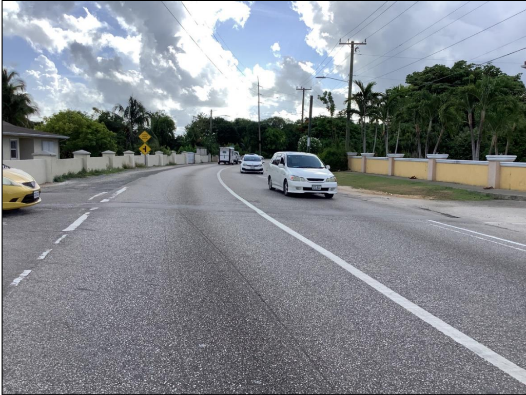
Photo 1: Two-lane road in residential area with relatively short decorative walls (July 2023)
