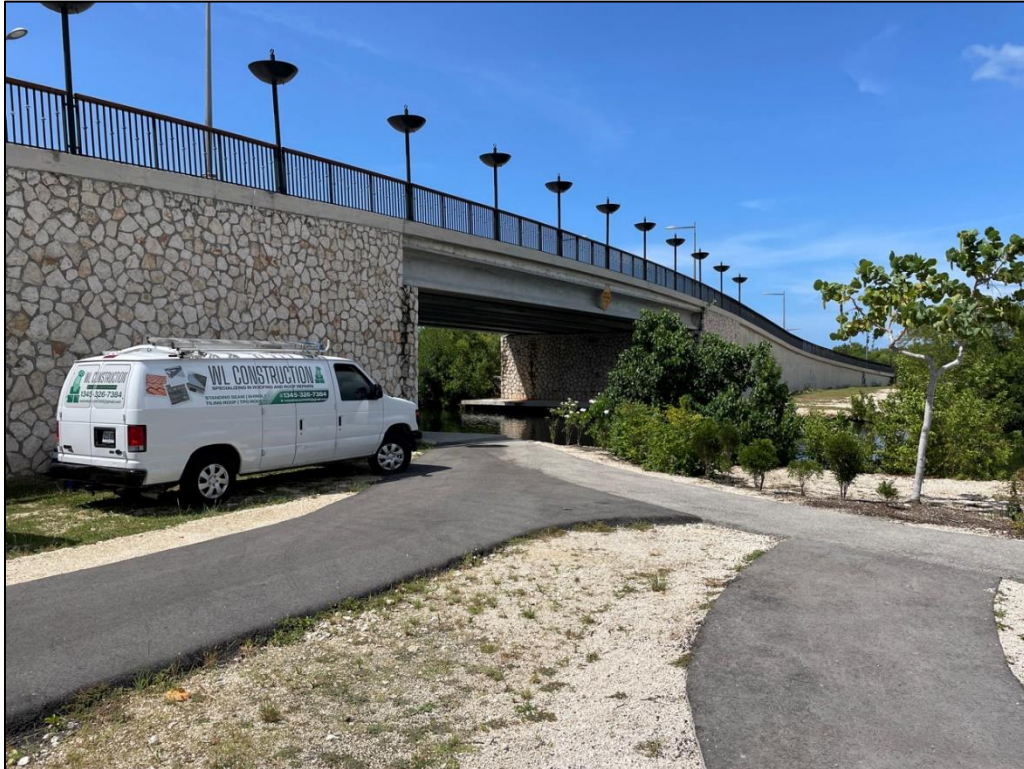
Photo 10: Existing Bridge in the Seven Mile Beach area (July 2023)
