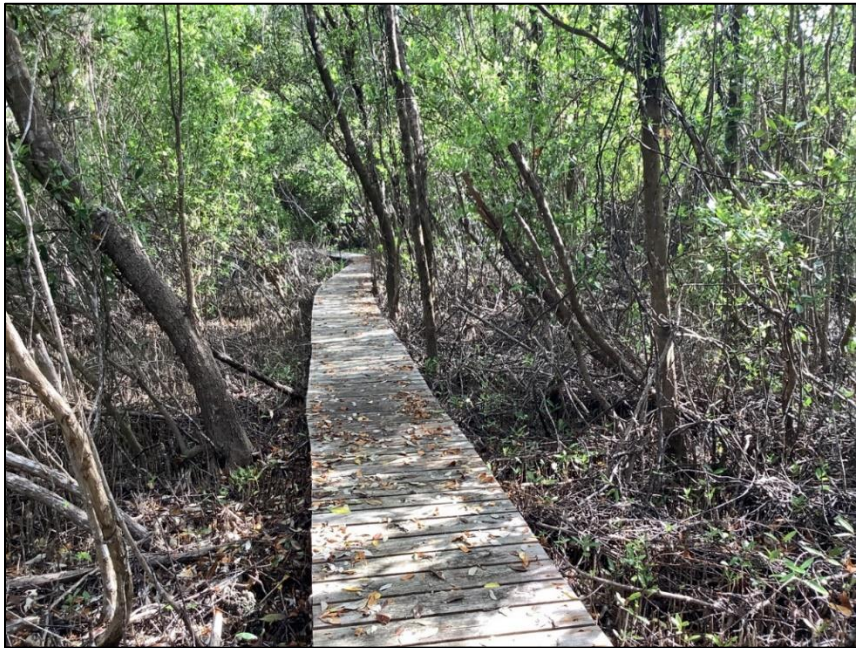
Figure 11: Mastic Trail – Boardwalk (July 2023)
