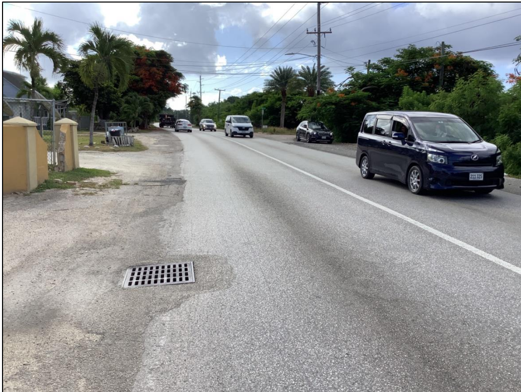
Photo 3: Typical inlet location (July 2023)
