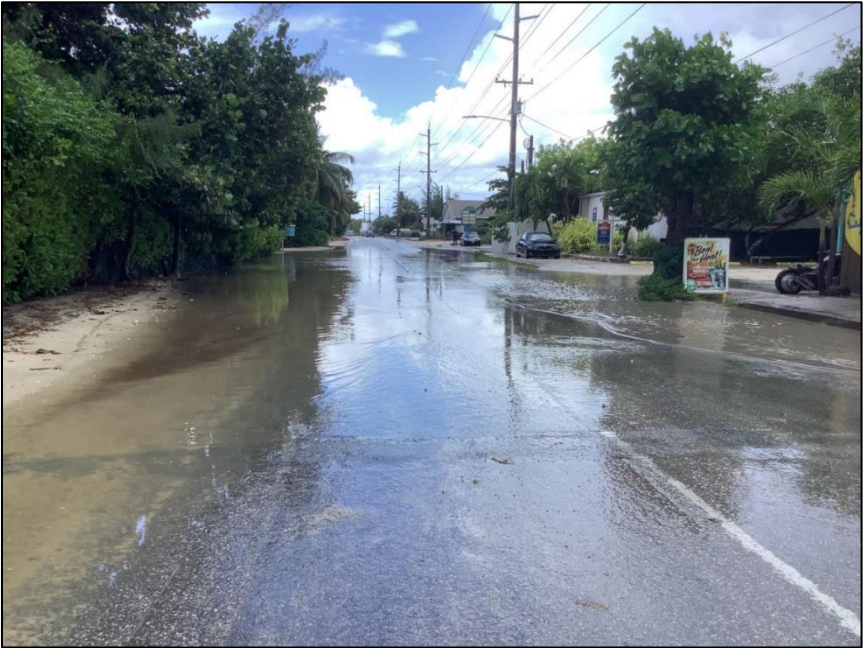
Photo 9: Flooding on Boddan Town Road after rainfall event (July 2023)
