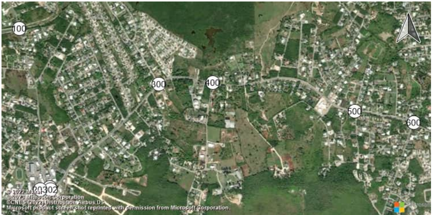
East-West Arterial at Hirst Rd Shamrock Road at Hirst Rd ( Shamrock Road at Hirst Rd ( Shamrock Road at Hirst Rd
