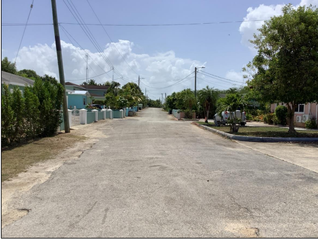
Photo 3: Unlined roadway in the proposed Will T Extension area (May 2024)
