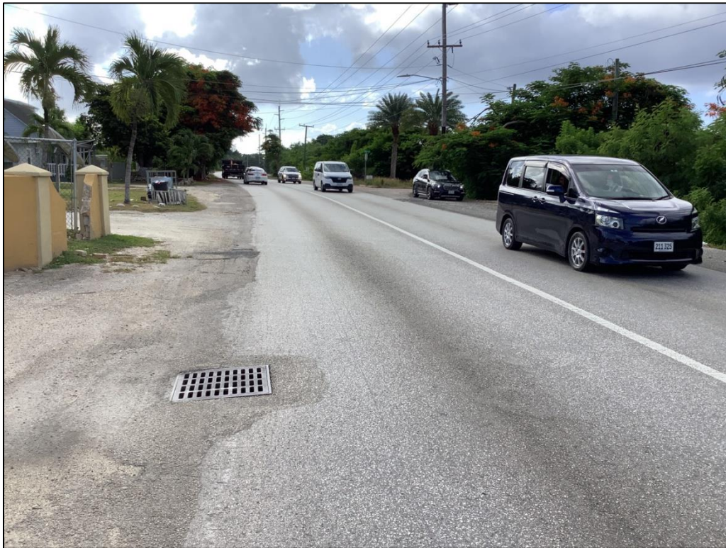
Photo 5: Typical inlet location (July 2023)
