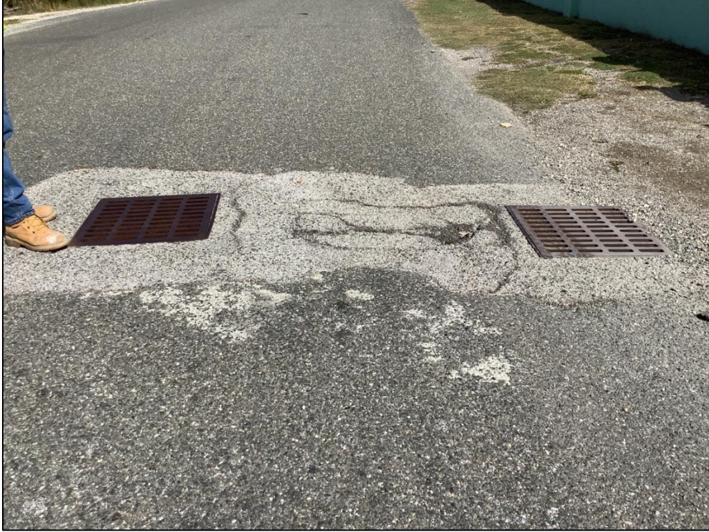
Photo 6: Inlet on shoulder drains to inlet in centre of roadway (July 2023)
