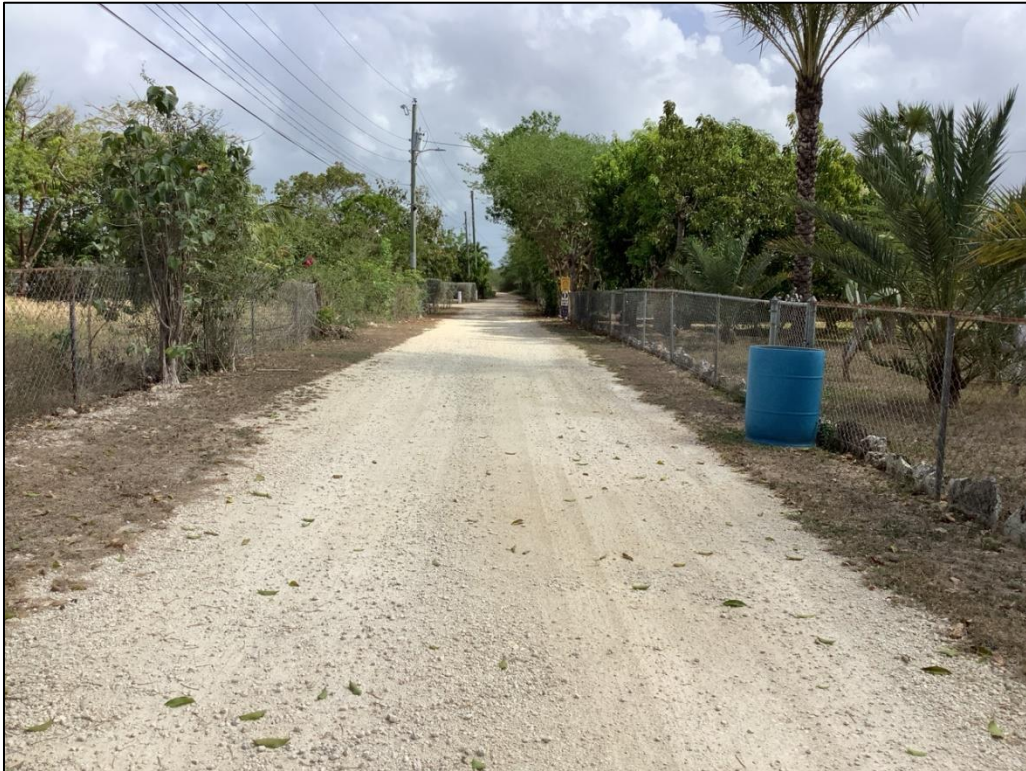
Photo 4: Trumbach Drive is gravel (May 2024)
