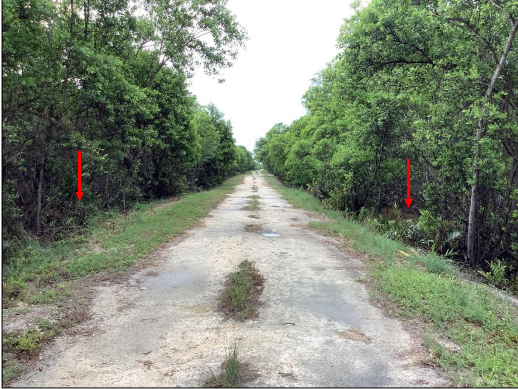
Photo 20: Access road with adjacent mosquito ditches (July 2023)
